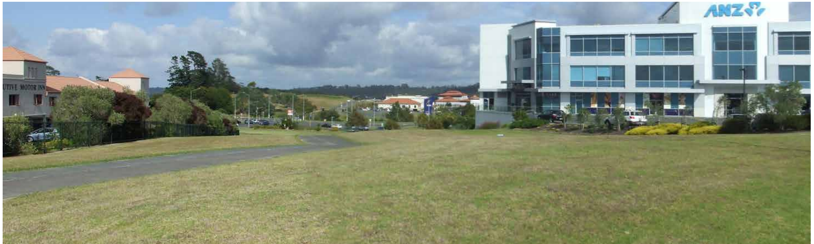
2. View looking southwest from Corinthian Drive, Albany
