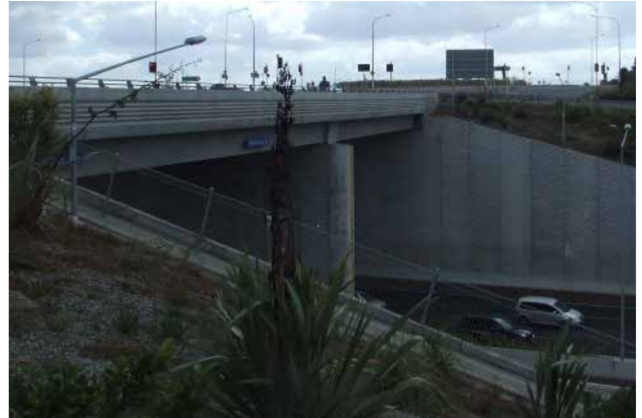
2. The corridor is heavily modified with few original natural elements remaining
