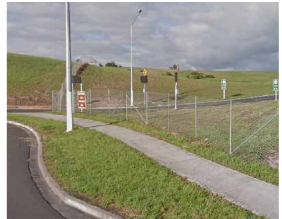
5. This photo was taken at the Brigham Creek Road intersection to show the infrastructural character of the receiving environment. Note the chain mesh fencing, light poles, signs and sealed surfaces.
