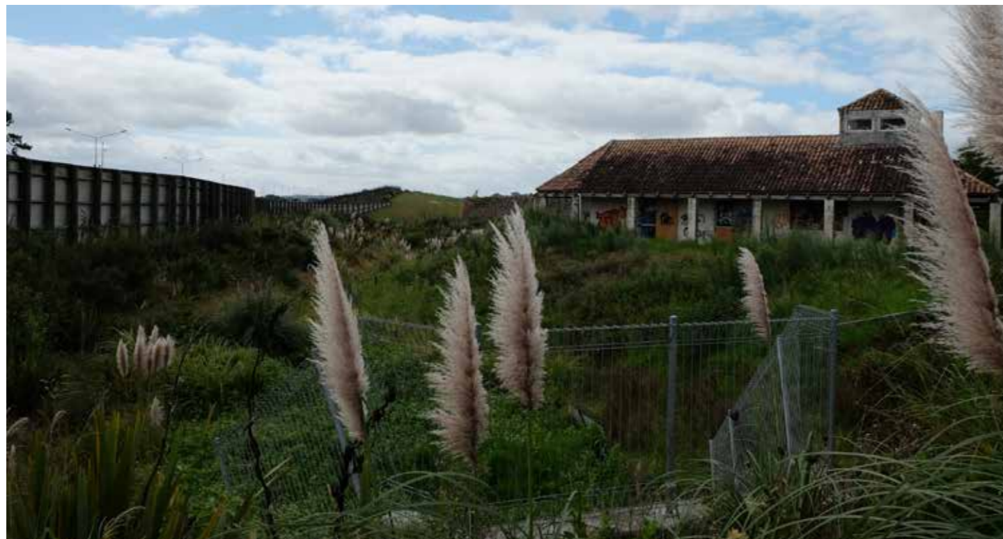
11. View from the entrance to 51 Trig Road towards the derelict house adjacent to the proposed MT8. The approximate 5m high motorway acoustic fence is to the left of the photo. Headwall structures are visible in the foreground.
