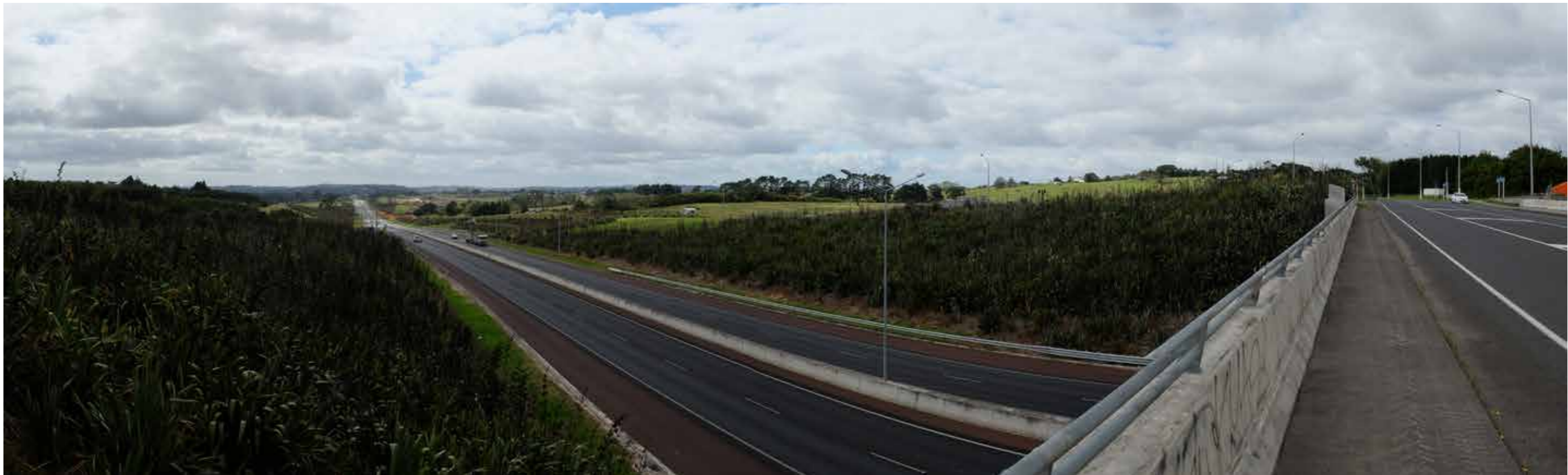
4. View looking north-east from Trig Road overpass
