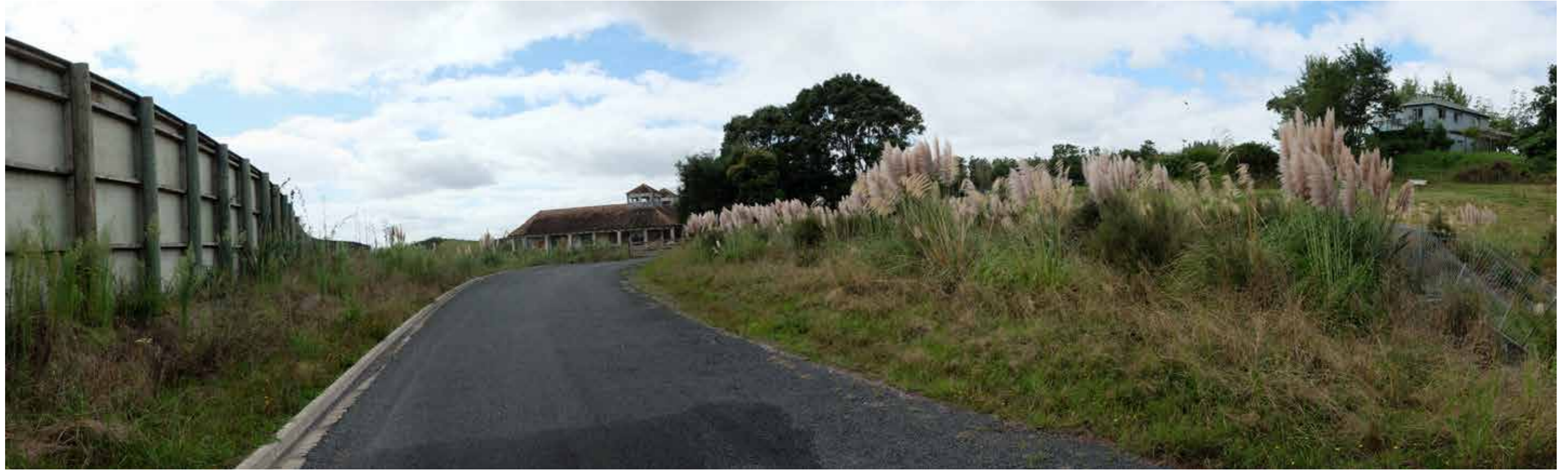
7. View looking east from the accessway to 51 Trig Road towards proposed MT8. The SH18 acoustic fence is on the left and existing dwelling to be demolished ahead.
