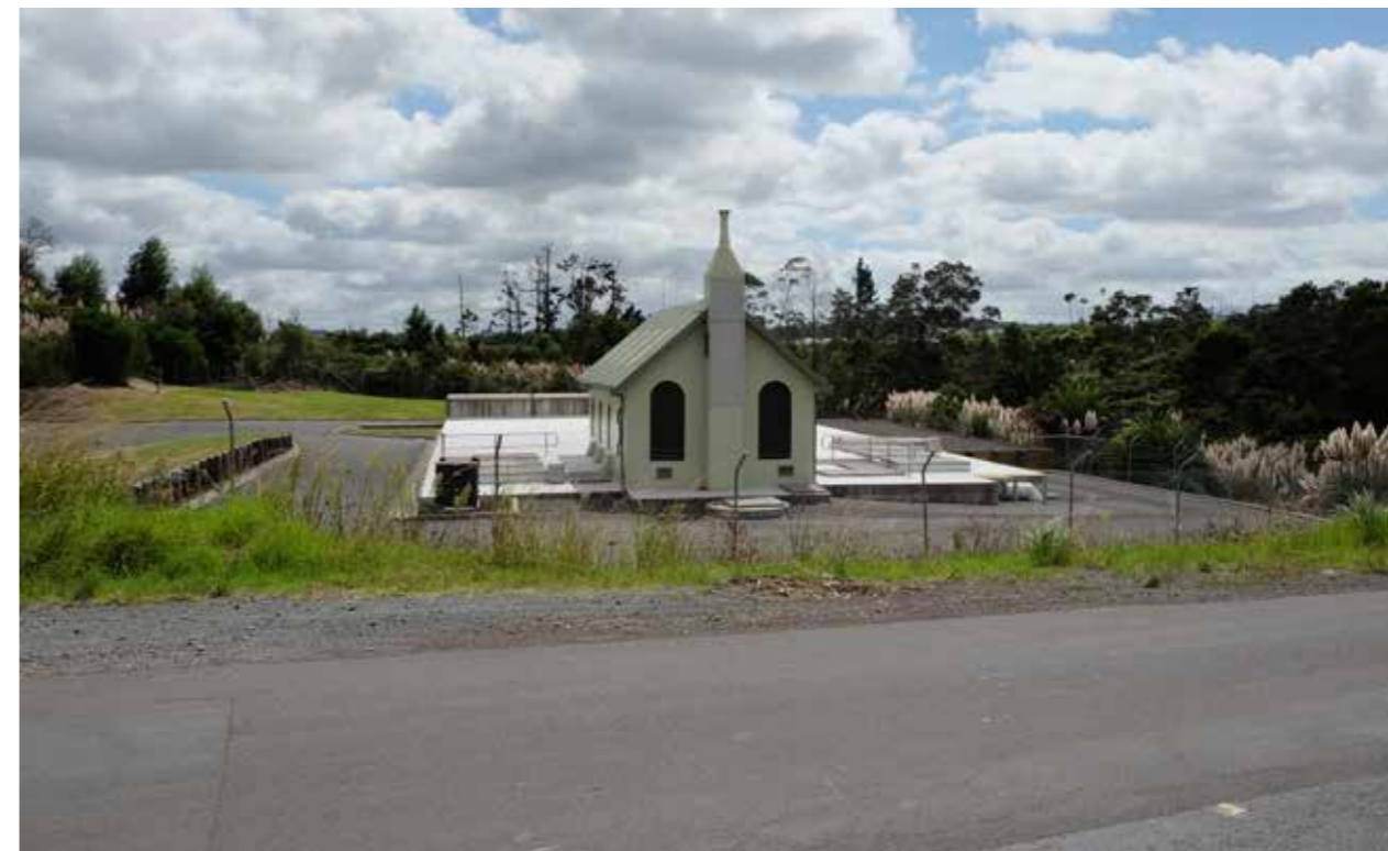
12. Pump house on Buckleys Road adjacent to MT17 and new Pump Station site.
