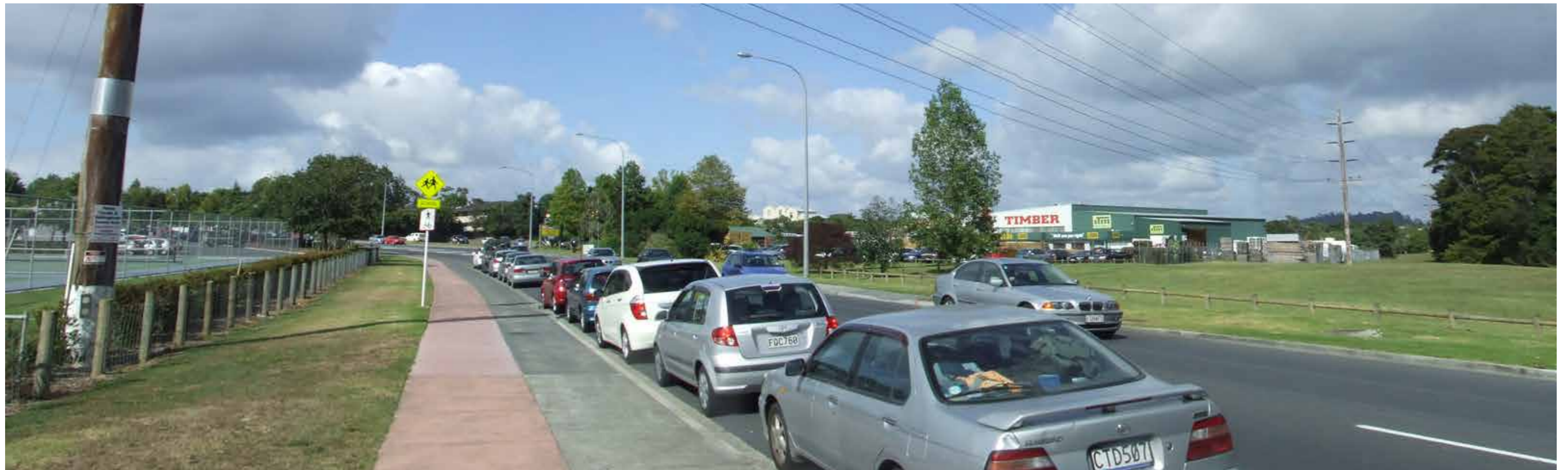
4. View looking southwest on Bush Road from Oteha Stream
